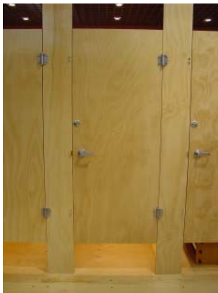
Blockboard doors used at a City Beach store, Brisbane.
